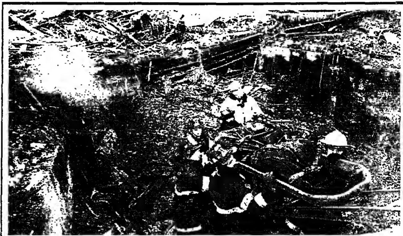
EXPLOSION IN CHICAGO — Fire fighters removing a victim from a collapsed building after blasts rocked residences and factories in Chicago. Caused by a faulty valve in a natural gas line, the blasts triggered 18 fires. Two persons were killed and five injured.
